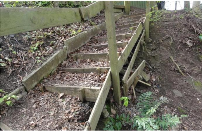
Peter is also planning to make some improvements to the steps and handrail, starting from the top, just behind Jim's container. Over time, the soil on the steep slope just below the steps tends to migrate downhill, which gradually undercuts the steps. He has a plan to improve the situation, but is going to carry out some trials before committing to the work.
